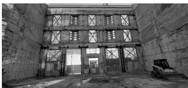
Figure 10. View from the interior of the construction site, from behind the supported historic façade
